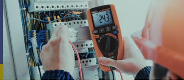
In residential installations, the CEI 64-8 standard requires certain checks in order to certify that the installation has been developed in a workmanlike manner. In addition to the usual voltage and current testers, HT ITALIA also offers simple, portable instruments for classic ground, RCD and insulation measurements.
